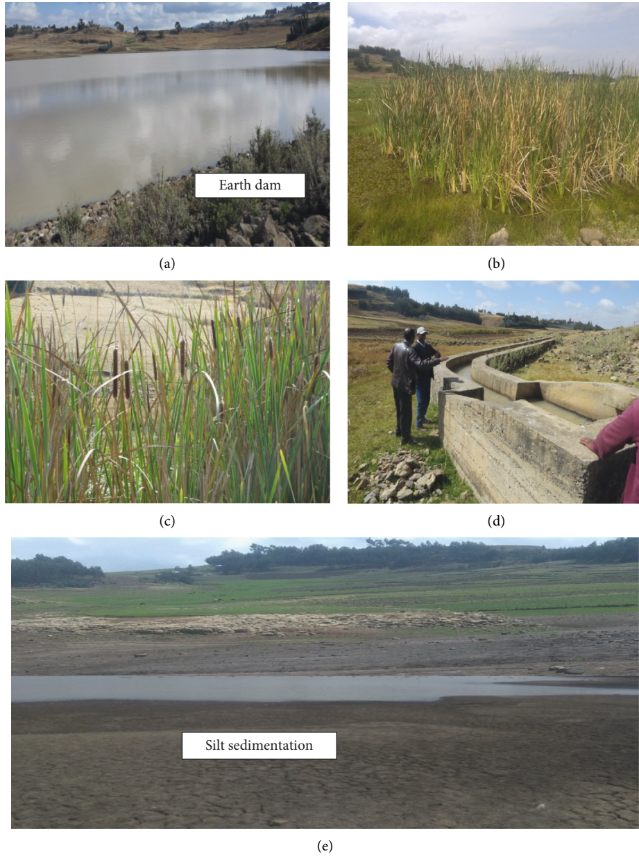
FIGURE 4: Partial views of Borale sites during the wet (a, b) and dry (c, d, e) seasons, with its reservoir and Earth dam (a), downstream wetlands covered with Typha , Cyperus , and Commelina species (b–c) and the canal (d), silt sedimentation, highly reduced water volume, catchment ploughed and covered with barely growing during a light rainy season (locally called ‘Belg’) from February to April and some woodlots of Eucalyptus globules nearby corrugated iron homes (e) (Photos taken from September 2020 to May 2021).
