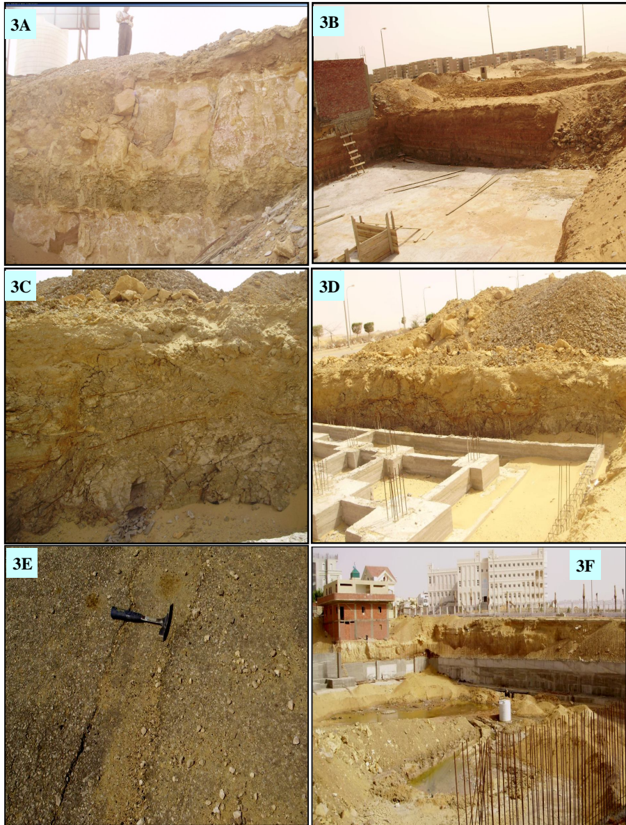
Fig.3: Showing some field Outcrop of Claystone beds (3B, 3C&3D), Sandy limestone bed (3A), Highway fractures (3E) and water flow under foundation beds (3F).
